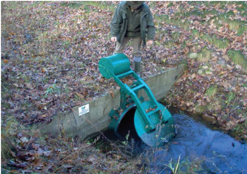
Figure. 3. A culvert with a backwater valve gate
