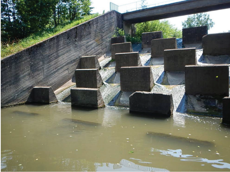
Figure 2. An example of interlocked-carpet block ramp (BR) of a Peterka kind constructed on Lubenia stream, phot. A.Radecki-Pawlik
