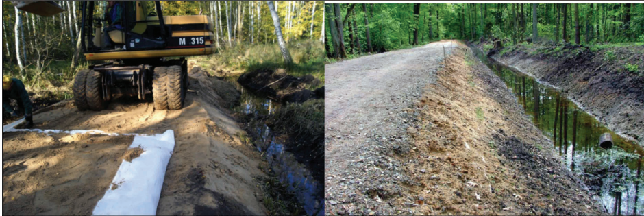
Photo 1. Construction of the experimental stretch of road (Photo A. Czerniak) and a view of the experimental stretch on the day of measurement (Photo S. M. Grajewski).
