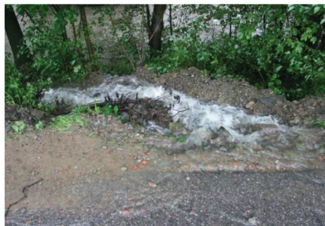
Photo 4. Intense surface runoff, erosion of channel banks and riverside infrastructure elements – September 2010 (source: commune archives)
