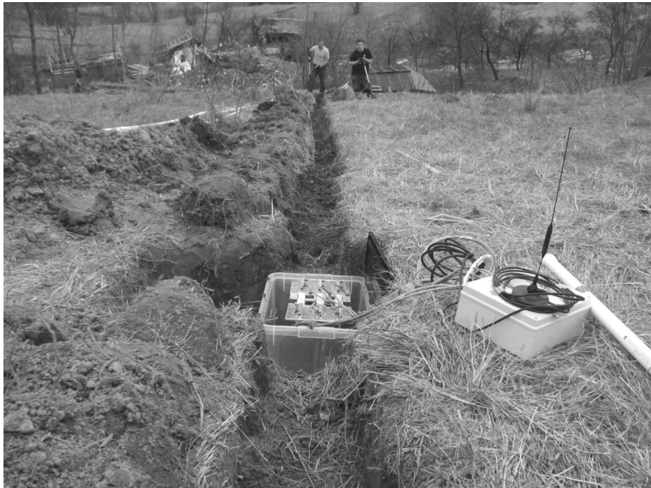
Figure 4. The field work
