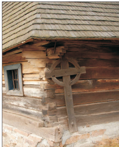
Phot. 105. Button-hole in swallow tale at a church in Bucea
