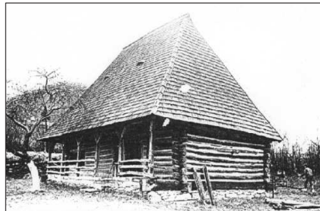
Phot. 104. House of joining beams - rounded button-hole
