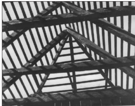
Phot. 107. Roof with rafter
