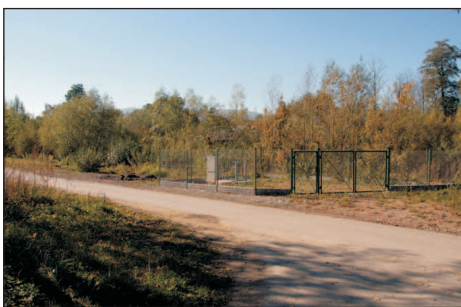
Phot. 30. Pumping station in Wiśniowa (photo: G. Kaczor)
