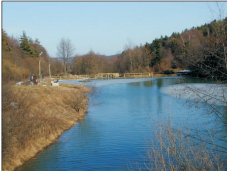
Phot. 17. Water intake from a small dam reservoir on the stream of Gościbia for the needs of water supply in Harbutowice (photo: G. Kaczor)
