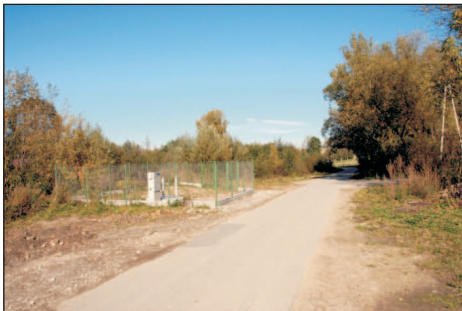
Phot. 39. Pumping station in Wiśniowa (photo: G. Kaczor)
