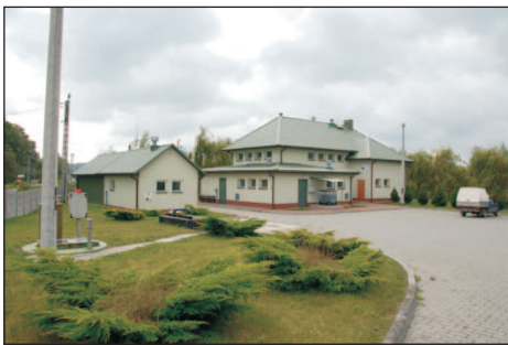
Phot. 28. Overall view of the sewage treatment plant in Książ Wielki (photo: G. Kaczor) (photo: G. Kaczor)
