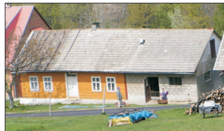
Phot. 65. A house with an attached building for livestock, after the latter has been converted into a brick structure. The building has retained its original shape. The wall of the house is covered with clapboards arranged horizontally and painted light brown (photo: W. Bieda)
