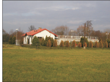
Phot. 27. Overall view of the sewage treatment plant in Kończyce Małe (photo: G. Kaczor)
