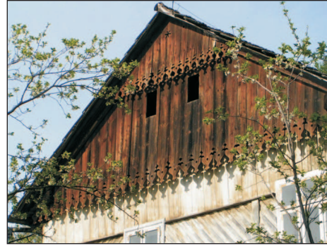
Phot. 53. A gable separated from the house wall with a double overhang covered with clapboards finished up with a decorative detail. The overhang casts a shadow on the wall, which duplicates the decorative detail (photo: W. Bieda)
