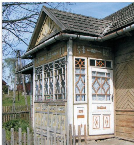
Phot. 56. A closed porch with large windows decoratively divided into smaller sections. Below, planks covered with geometric shapes. In the upper part, planks are covered with different patterns, including plant-like motifs. The tympanum of the porch is decorated with a carved barge board and a radial ornament called 'słonecko' borrowed from the architecture of the Podhale region (photo: P. Herbut)
