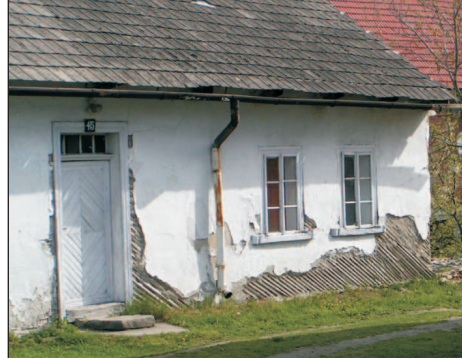
Phot. 45. A fragment of a wooden house with the ground floor almost at the ground level: walls plastered with clay laid on wooden slats; the entrance door covered with decoratively arranged clapboards and a transom window (photo: W. Bieda)
