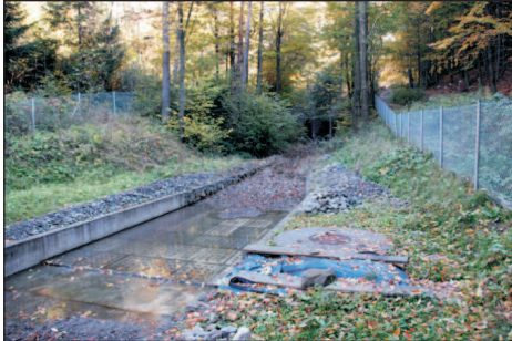
Phot. 31. Water intake on the Na Padoly stream (photo G. Kaczor)
