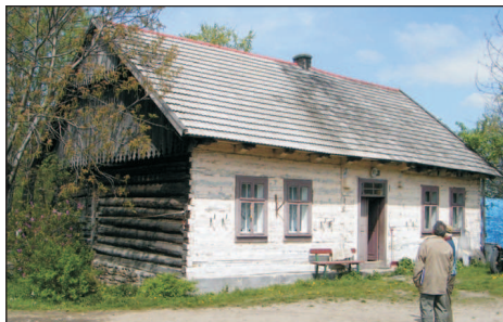
Phot. 48. A house plastered with clay and whitewashed with lime - only at the front (photo: P. Herbut)
