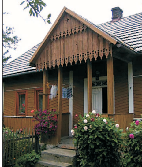
Phot. 59. An open porch, supported by 4 poles: a balustrade at the sides fully covered with clapboards; the tympanum with overhang clapboards finished up with elaborate details and an opening in the shape of a cross (photo: P. Herbut)
