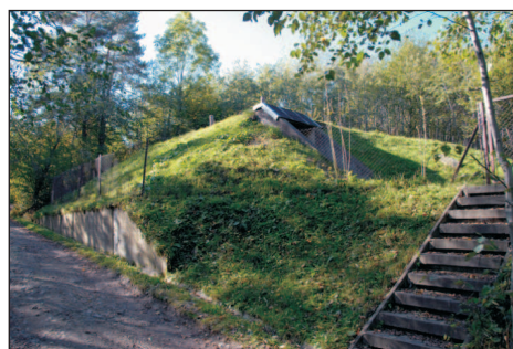
Phot. 36. Ground water reservoir in Lipnik (photo: G. Kaczor)
