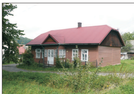
Phot. 43. A house built in the years 1947/48 with a half-hipped roof: after the change of roof covering, the tympanum was separated from the wall with a narrow roof (photo: P. Herbut)
