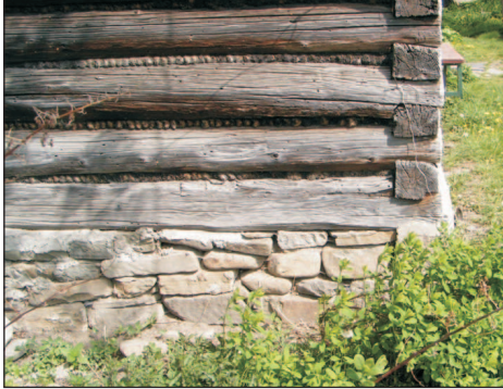
Phot. 44. A fragment of a wooden house from the end of the 19th century: a corner-notched log wall laid on a shallow stone foundation with clay mortar; a dove-tail joint. Empty spaces between beams filled with moss and tails of straw (photo: W. Bieda)
