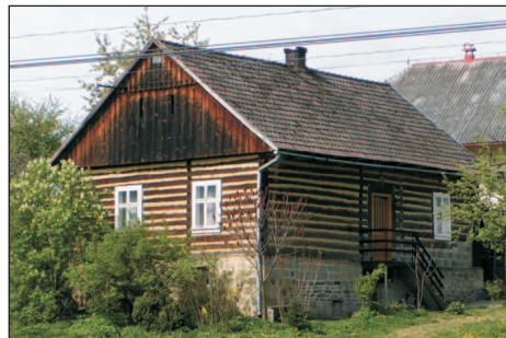
Phot. 47. A house on a high stone underpinning: gaps between beams filled with clay; the southern gable has a natural colour of 'old' wood with brighter stripes along the eaves and under the upper clapboard overhang (photo: P. Herbut)
