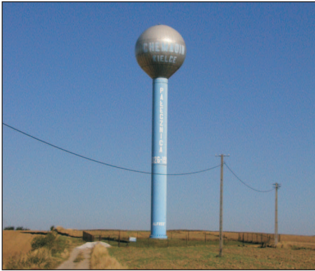
Phot. 22. Tower reservoir in the community of Pałecznic (photo: G. Kaczor)
