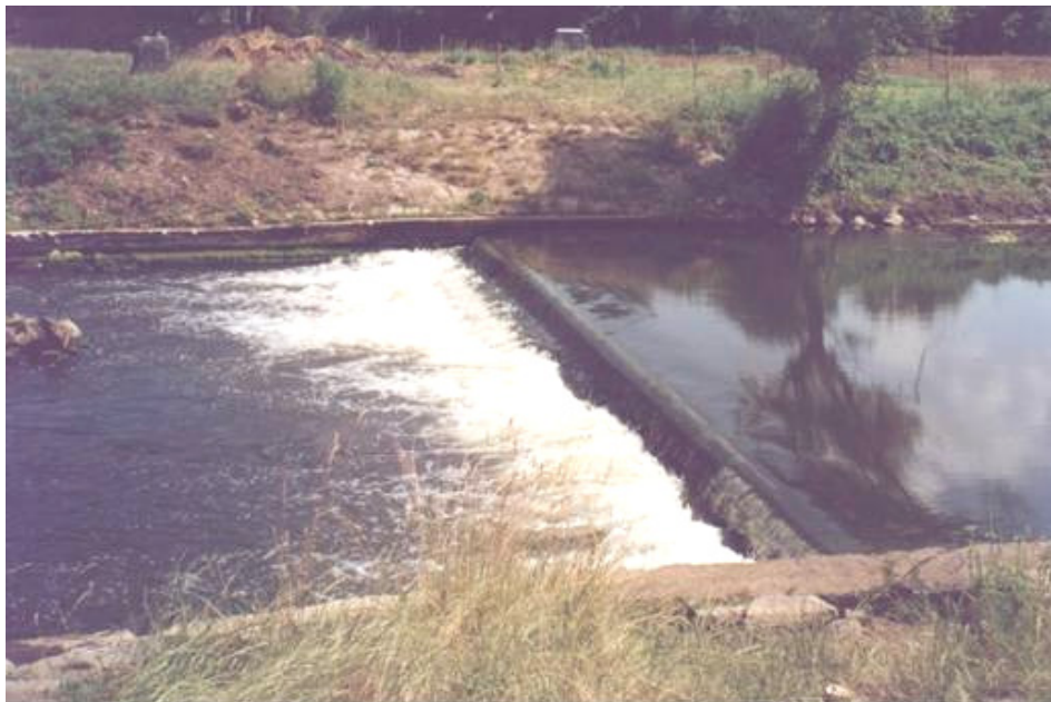
Fotografia 1. Jaz Widawa Polanowice km 12+435 Photo 1. Widawa Polanowice weir on 12+435 river kilometer
