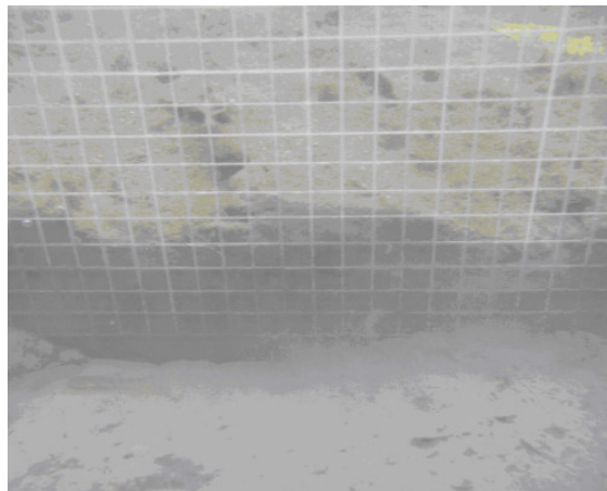
Figure 5. The profile of the bottom of the Krempna reservoir made in the inlet cross-section (cross-section II)
