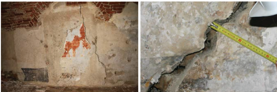
Figure 4. A view of exemplary cracks recorded during inventory
