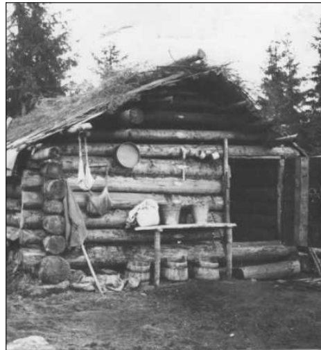
Phot. 106. Semi-cylindrical coronet roof in a sheepfold
