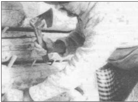
Phot. 108. Fixing the plaster
