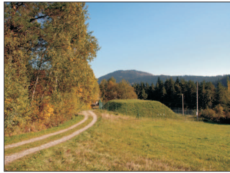
Phot. 34. Ground water reservoir in Kobielnik (photo: G. Kaczor)
