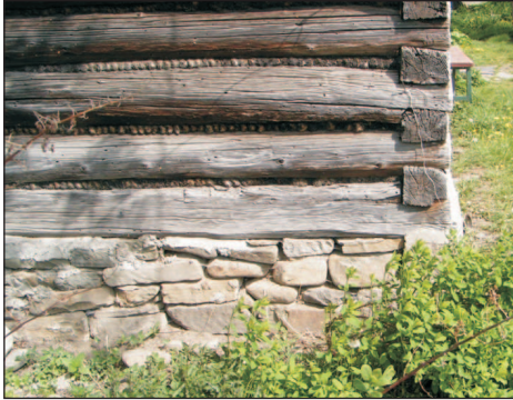
Phot. 44. A fragment of a wooden house from the end of the 19th century: a corner-notched log wall laid on a shallow stone foundation with clay mortar; a dove-tail joint. Empty spaces between beams filled with moss and tails of straw (photo: W. Bieda)
