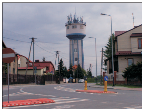
Phot. 25. Tower water reservoir in Kraków - the district of Skotniki (photo: J. Pawełek)
