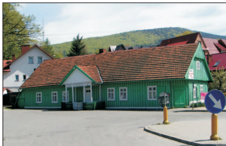
Phot. 62. The house of the organist build at the end of the 19th century: an open porch supported by 4 poles; a characteristic tympanum with a rare double ornamented detail (the so-called ‘fartuszek’); window frames, the porch tympanum and vertical slats covering clapboard contact points, all painted white, contrast with green walls and shutters (photo: W. Bieda)
