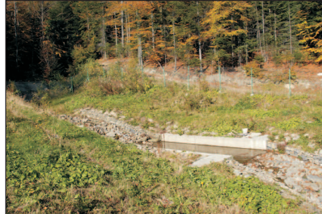
Phot. 32. Surface water intake on the Smarkawa stream (photo: G. Kaczor)
