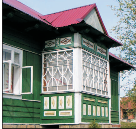
Phot. 55. A closed porch with edges and window frames painted white, strongly contrasting with green walls. Below decoratively divided windows, planks covered with rhombuses and rectangles. In the upper part, the planks have different colours and patterns (photo: P. Herbut)
