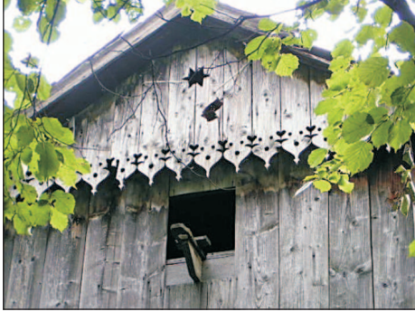
Phot. 54. A fragment of a gable with a beautifully patterned architectural detail: a star-shaped opening and a larger opening with a small balcony for pigeons (photo: W. Bieda)
