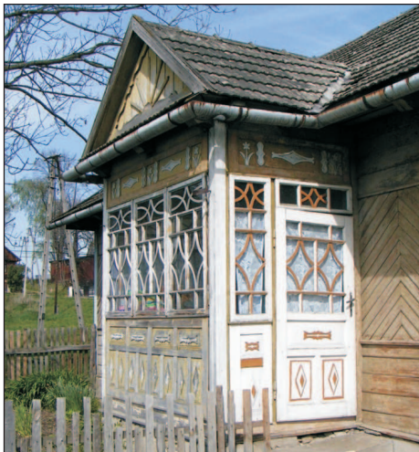
Phot. 56. A closed porch with large windows decoratively divided into smaller sections. Below, planks covered with geometric shapes. In the upper part, planks are covered with different patterns, including plant-like motifs. The tympanum of the porch is decorated with a carved barge board and a radial ornament called 'słonecko' borrowed from the architecture of the Podhale region (photo: P. Herbut)
