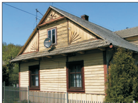
Phot. 61. A gable with two small roofs: a carved slat running along the eaves and a radial ornament - elements typical for the architecture of the Podhale region. New windows on the ground floor correspond to traditional patterns (photo: P. Herbut)
