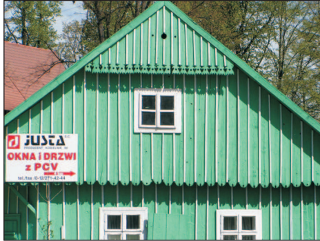
Phot. 52. A gable with a double overhang covered with clapboards finished up with variously decorated details. The shadow on the wall highlights the overhang (photo: W. Bieda)
