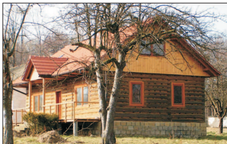
Phot. 66. A house on a stone underpinning being adapted for a holiday cottage: an open porch supported by 2 poles has been added; roof covering and window frames have been exchanged. New windows do not retain the traditional pattern while the window in the gable strikes with excessive size (photo: P. Herbut)
