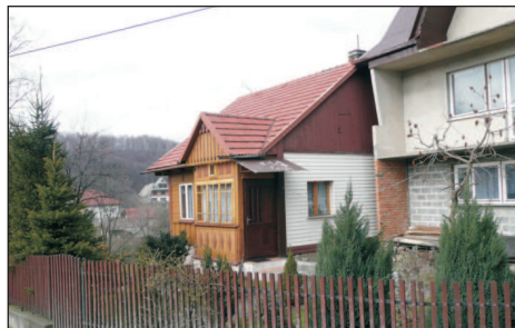
Phot. 67. A house with a beautiful porch, partially taken down to make space for a new building (photo: W. Bieda)
