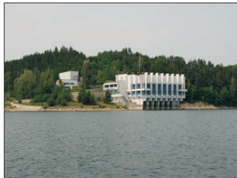
Phot. 18. A water intake from the Dobczyce reservoir for the needs of Krakow (photo: G. Kaczor)
