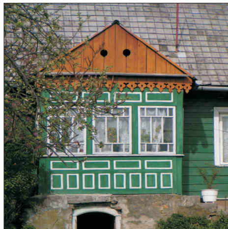
Phot. 57. A spacious, closed porch with a cellar: large windows with characteristic division into squares and rectangles; similar patterns placed on planks on porch walls; white window sashes and planks strongly contrast with green walls; the tympanum finished up with decorative details (photo: P. Herbut)
