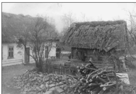
Phot. 42. The year 1970, Na Sodku, the oldest farm in Wiśniowa; a house and a building for livestock with double-pitched thatched roofs (from the Kronika Szkoły Podstawowej w Wiśniowej of 1970)
