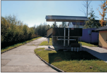
Phot. 37. Sewage treatment plant in Wiśniowa (photo: G. Kaczor)
