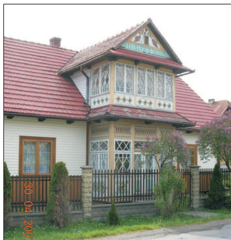
Phot. 51. A house raised in 1935, currently after thermal modernisation: the walls covered with shining siding; the porch with a dormer window; everything richly decorated; large glazed surfaces decoratively divided into smaller parts; new windows are suitable in terms of size and their structure corresponds to traditional patterns (photo: P. Herbut)
