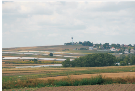
Phot. 23. Location of a tower reservoir in Kocmyrzów-Luborzycza (photo: G. Kaczor)
