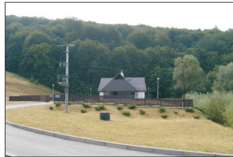
Phot. 29. A general view of the sewage treatment plant in Żary (photo: A. Chudecka)
