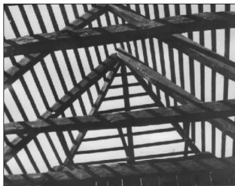
Phot. 107. Roof with rafter
